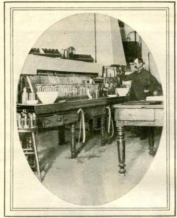
IN THE ASSAY OFFICE—BOILING SAMPLES OF GOLD IN NITRIC ACID, TO DISSOLVE THE SILVER WITH WHICH THE GOLD IS USUALLY ALLOYED.
