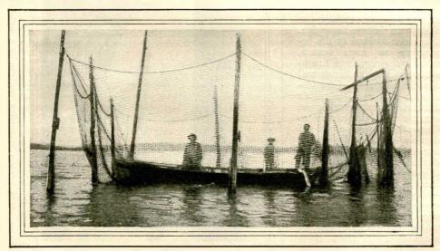
THE "POT" OF A COLUMBIA RIVER SALMON TRAP, SHOWING HOW THE NET THAT FORMS THE BOTTOM
